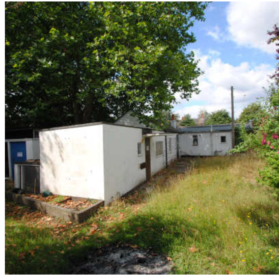
External view from east
